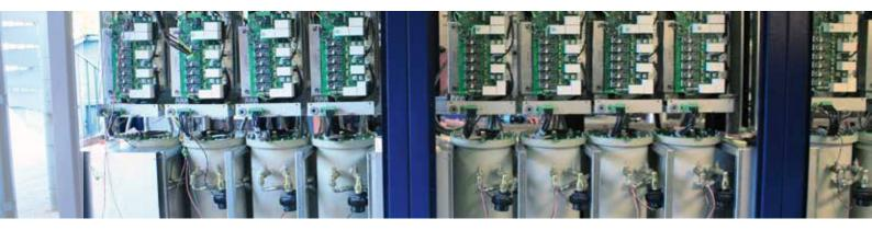
Using SMPS technology to energize electrostatic precipitators enhances both total collection efficiency and fine particulate collection. This is achieved mainly due to the almost ripple-free high voltage signal provided by a high frequency power supply, where a traditional Transformer/Rectifier (T/R) will have a ripple similar to the low frequency - 50/60 hz - of the mains input.
