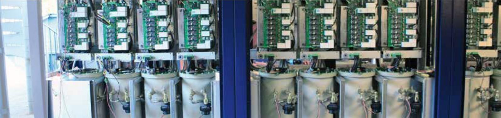
Using SMPS technology to energize electrostatic precipitators enhances both total collection efficiency and fine particulate collection. This is achieved mainly due to the almost ripple-free high voltage signal provided by a high frequency power supply, where a traditional Transformer/Rectifier (T/R) will have a ripple similar to the low frequency - 50/60 hz - of the mains input.
