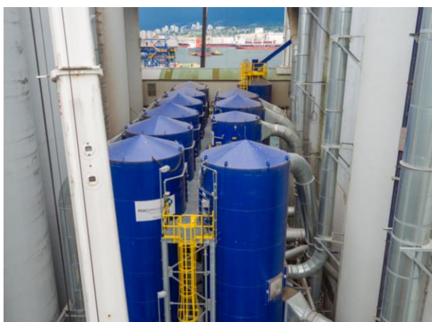
Viterra installed MCF Powersaver® dust collection systems at two grain processing terminals to improve their dust collection process.
