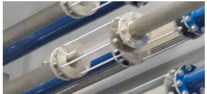
Pneumatic conveying pipe lines
