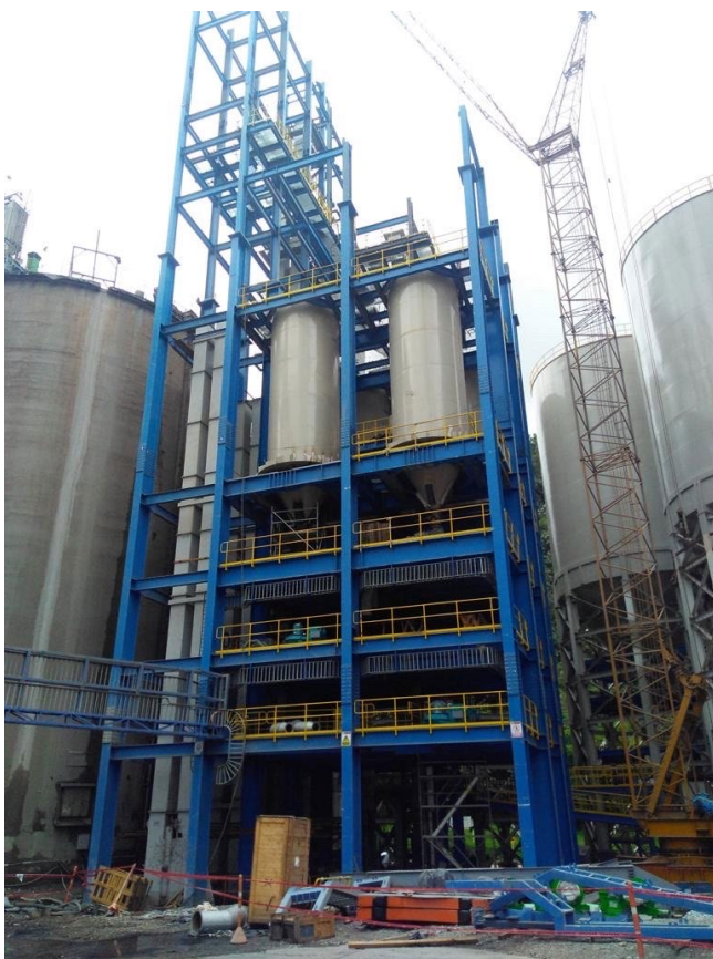
Installation of blending system at Argos Rio Claro
