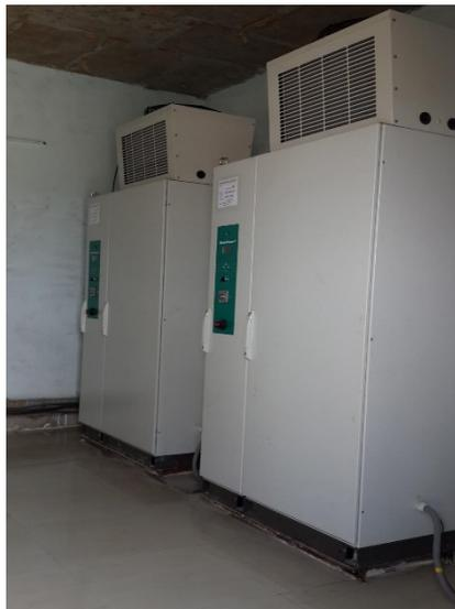
**Fig- 2: 2 x 60 kW ModuPower™ TM MPX cabinets mounted remotely in control room. 100kV rated HV cable used to connect MPX to ESP**
