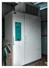
Figure 4: 1 x 60 kW ModuPower™ MPX cabinets mounted in ESP rooftop. 100kV rated HV cable used to connect MPX to ESP
