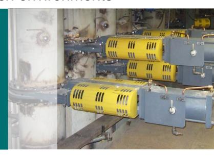
KGVs are designed to handle high velocity material dust contamination, limited maintenance access, and infrequent valve operation. These valves will maintain operational integrity after continuous exposure to internal flow of high velocity material and air mixture. KGVs meet the NFPA requirements for containment of explosion pressures.
