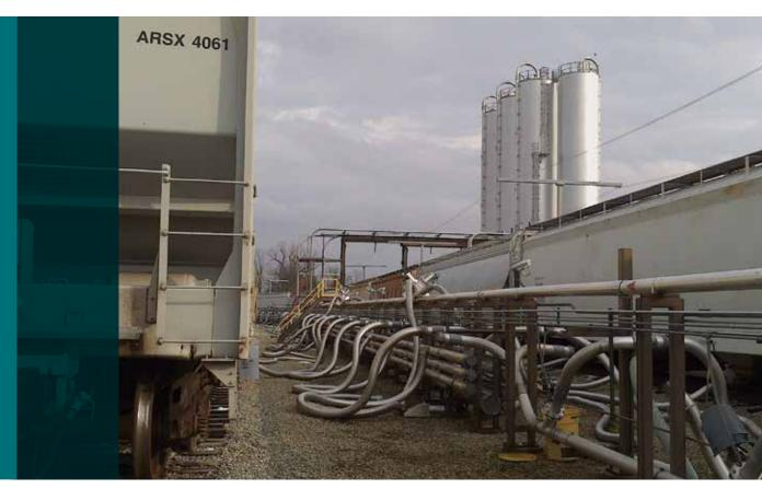
For the efficient unloading of railcars or trucks in plastics processing applications, Schenck Process pneumatic conveying systems are the right choice for handling incoming bulk solid materials and transferring them into your plant process.
